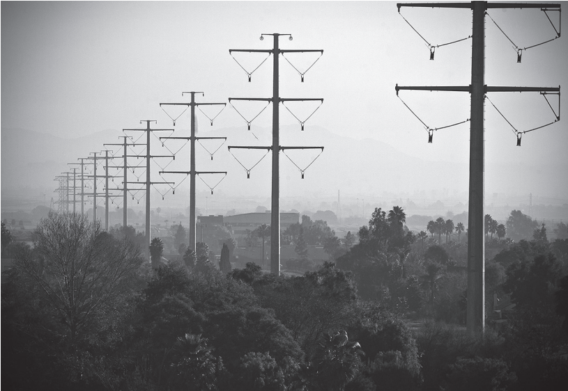
2. Steel towers for 500kV transmission line in Chino Hills, California, 2014. The 198-foot towers formed a segment of the Tehachapi Renewable Transmission Project. A court order later forced Southern California Edison to remove the towers and run this section of the 500kV line underground. Photo by Thomas Cordova.
