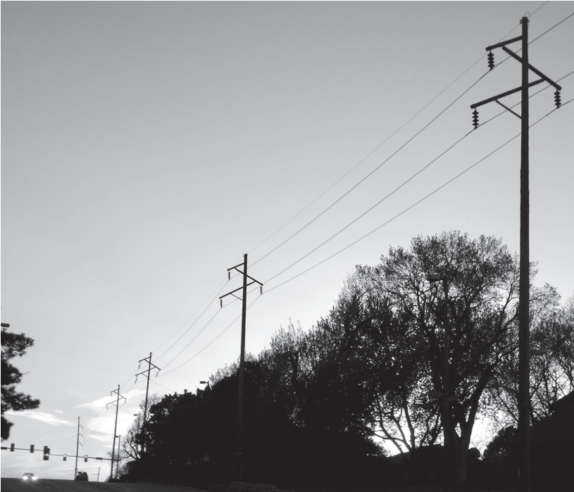
1. 69kV transmission line, 2018. The three slanted arms attached to the pole form what some utility line workers call a “wishbone” configuration. I began the imaginary “power lines” game at this corner of Blondo and 102nd Street in Omaha, Nebraska. Photo by Eva Hernandez.
